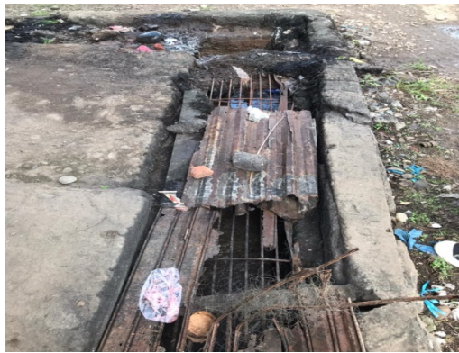
Drainase Pasar Barukoto
